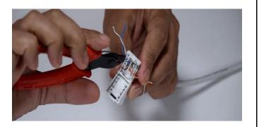
Step 2: Cut off unwanted cable protrusions.
